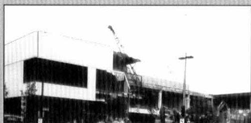
Out with the old - in with the new!! The old MECCA center, home of GENCON in years past is demolished.
